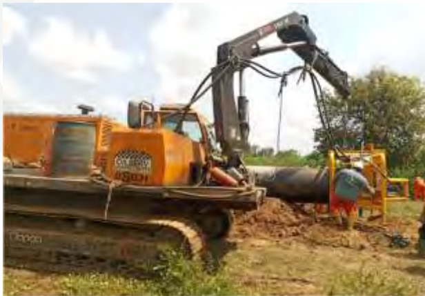
Automatic Welding Machine in action at site for AKK project
