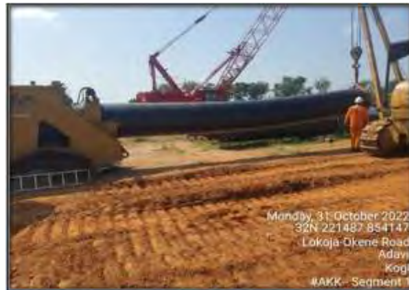
Cold Bending in progress at site for AKK project
