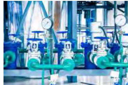
Water re-injection platform of Produced Water Disposal
