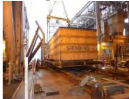
Compressor installation
